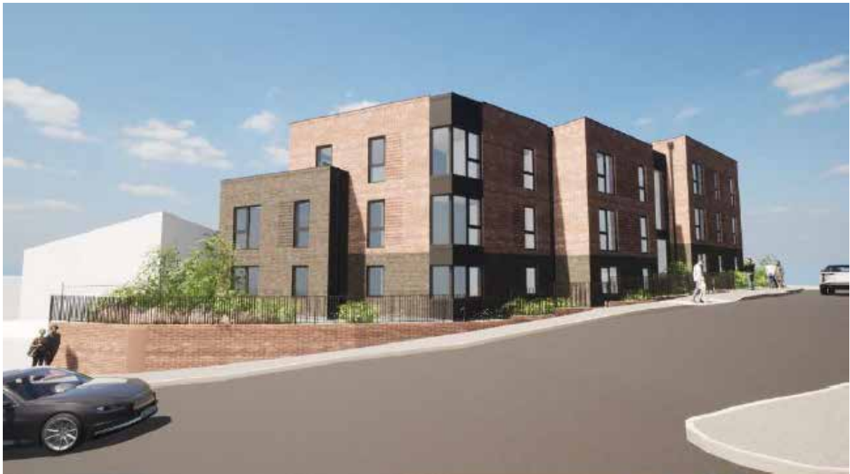
Corner elevation fronting Kelham Way junction
